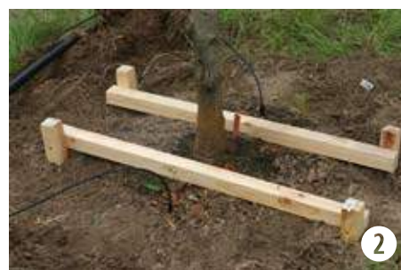
Figure 2 Root ball anchorage systems work nicely.
