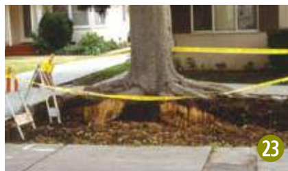
Figure 23 Construction is especially damaging to roots, such as these roots cut during curb repair.
