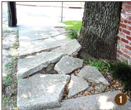
Figure 1 Sidewalk located too close to the root flare of a large tree.
