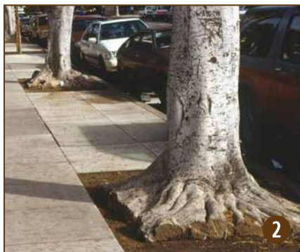
Figure 2 Main supporting roots were cut. These trees, once of value to the landscape, are now at high risk for failure and should be removed before they fall over.
