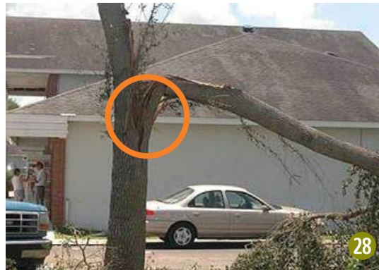
Figure 28 This tree should be removed since its broken stem is very large and the trunk is cracked, as shown by the circle. If the tree were not cracked into the trunk, the broken limb could be carefully removed and the tree might be restorable.
