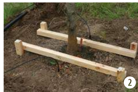
Figure 2 Root ball anchorage systems work nicely.
